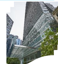
Menara 3 PETRONAS – Retail Podium
