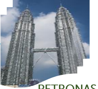
PETRONAS TWIN TOWERS
