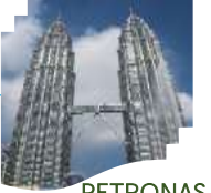
PETRONAS TWIN TOWERS
